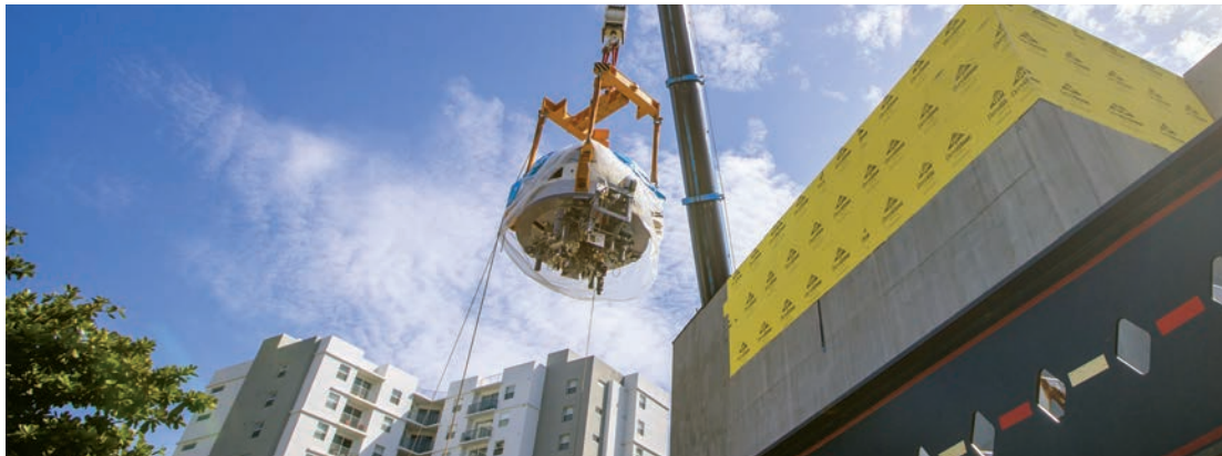
Cyclotron installation through Sylvester's roof.
